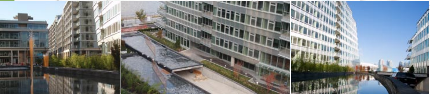
Inset series, left: Reflecting ponds at Parcel 4 add beauty and intrigue to the structure’s design – and serve the functional purpose of circulating stored rainwater to ensure it stays clean. The water in the ponds thus does not require chlorination, giving the option of adding aquatic plants if desired.
