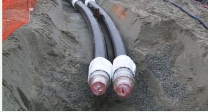
A distribution pipe system runs beneath the streets at SEFC, delivering thermal energy in the form of heated water from the Energy Centre to each of the buildings. Pipes are well insulated in order to reduce or eliminate energy loss through the distribution process.
