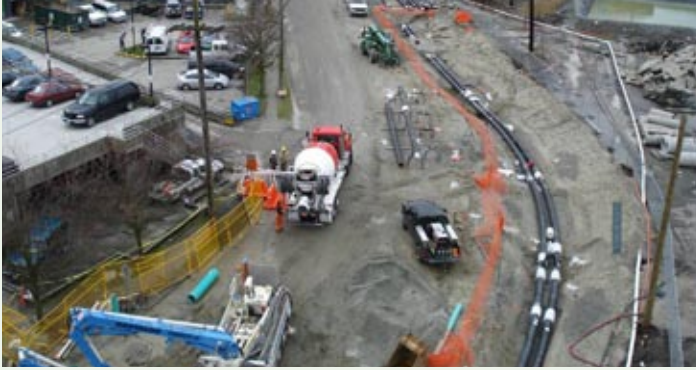
A distribution pipe system runs beneath the streets at SEFC, delivering thermal energy in the form of heated water from the Energy Centre to each of the buildings. Pipes are well insulated in order to reduce or eliminate energy loss through the distribution process.
