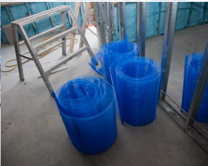
The capillary mat heating system is made of polypropylene, making it easy to repair (though tenants are reminded not to puncture the ceiling!). Hidden from sun damage, they are extremely durable and long-lasting.
