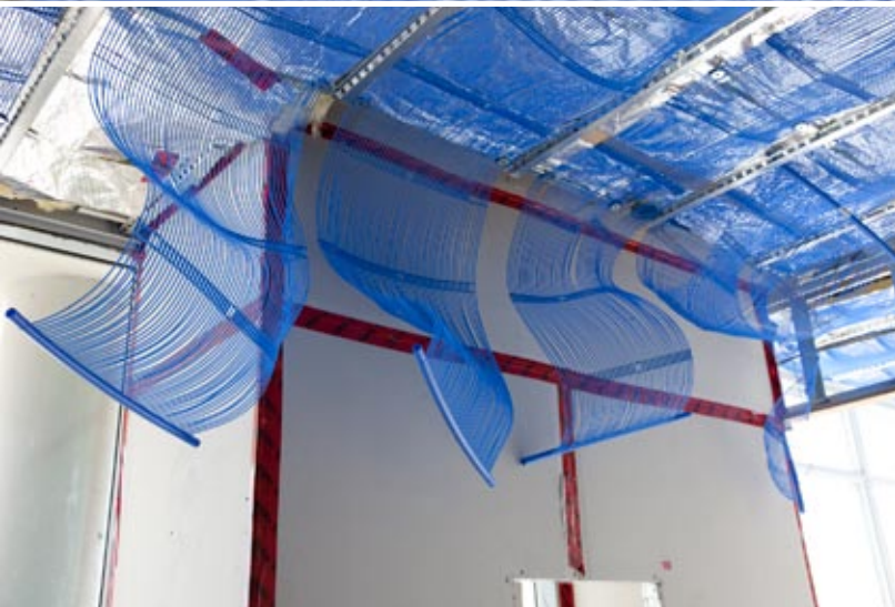
The capillary mat heating system is made of polypropylene, making it easy to repair (though tenants are reminded not to puncture the ceiling!). Hidden from sun damage, they are extremely durable and long-lasting.
