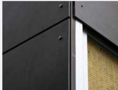
SWISSPEARL • Fibre reinforced cement panel available in wide variety of colours • Durable, low-maintenance
