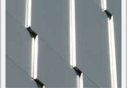
ALUCOBOND, REYNOBOND • Metal composite sheet materials with durable finishes • Can be shaped to suit varied architectural applications • Low maintenance
