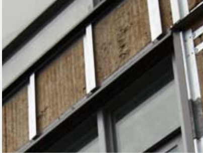
ROCK + SLAG MINERAL WOOL INSULATION (ROXUL) • Manufactured in BC • Consists of basalt rock and recycled Steel slag, with a minimum 40% recycled content
