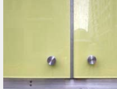
FRITTED GLASS • Glass with enamel image fired onto surface • Allows durable colour options
