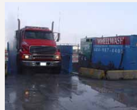
Middle and bottom: Wheel-wash stations remove contaminants from all truck wheels before they leave the site.
