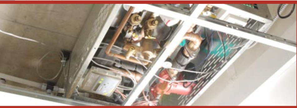
Above, Energy Centres are installed in the ceiling of each suite. Background, a detailed layout diagram for installation of the capillary mat system. “Our company got very deeply involved in the design and layout of the ceilings,” says Peter MacLellan of Olympic International. “We needed to make everything as simple as possible, to not leave any guesswork.”
