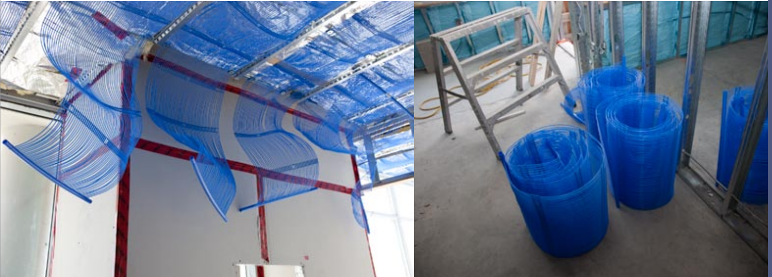
The capillary mat heating system is made of polypropylene, making it easy to repair (though tenants are reminded not to puncture the ceiling!). Hidden from sun damage, they are extremely durable and long-lasting.
