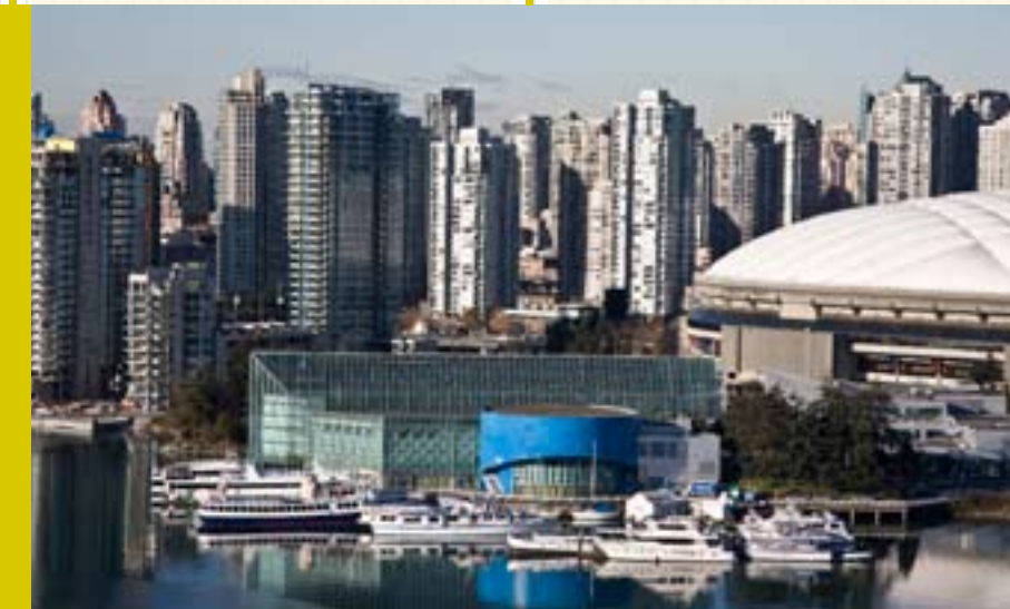
False Creek North boasts high-density, high-rise residential living and community amenities. SEFC's unique approach demonstrates a shift to low- and mid-rise density with a focus on environmental and community benefits.
